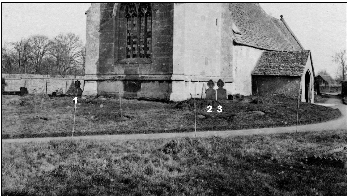
Plate ii. A second 1884 view of the church and churchyard looking north-east, showing the 'Hamble' family monument (1), and the 'Warmington' and 'Parker' monuments (2 & 3). These three monuments are still in the same locations, but the 'Hamble' monument is now lying flat. The kerb stones surrounding the plot shown in the lower right hand corner of this photograph were not found during this survey, and were probably removed in the 1940s when this area was reused for new burials.
