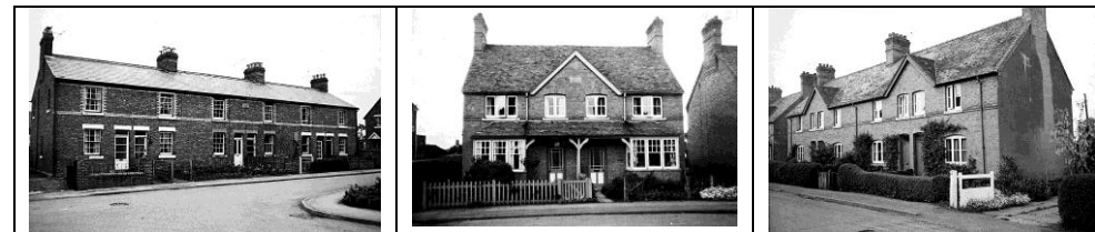
Houses on the north side of Brewers Lane, built 1893-1903, taken in 1968 by Birmingham Photographic Club: 13-23 (South View Terrace); 33-35 (Tower View); 37-43 (Fair View).
