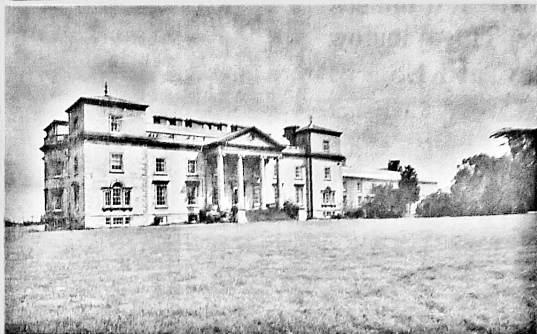
Croome Court, in its 38 acres of grounds landscaped by Capability Brown, has been sold by the Trustees of the Bedford Court and Croome Residential Special Schools to a London agent acting for the proprietors of a preparatory school. Locke and England, who handled the sale for the vendors, say the price was more than £300,000. The house was built in 1752 for Lord Coventry.
