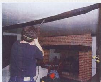
Photo 3: Extraction of a core in progress
