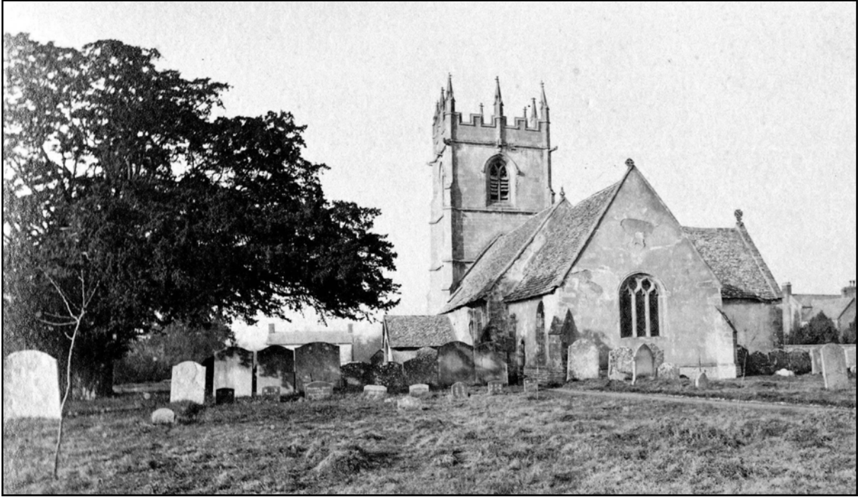
Plate i. View of Badsey church and churchyard looking south-west. This photograph, taken in 1884, shows headstones with accompanying footstones. Most of these footstones have not been found during this survey. All headstones shown are now lying flat in the grass; some face down with the inscribed faces totally eroded.
