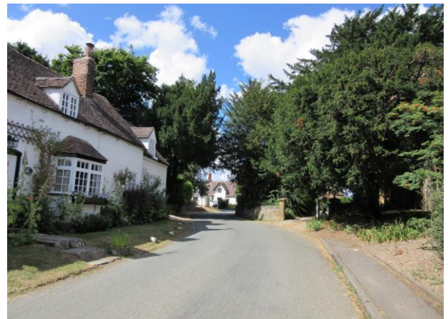
Continuing north along Village Street, views are afforded of Corner Cottage
