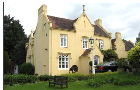
Aldington Lodge – knocked down to make way for new housing on Lodge Park Drive. Photo Gill Stewart, 2008.
