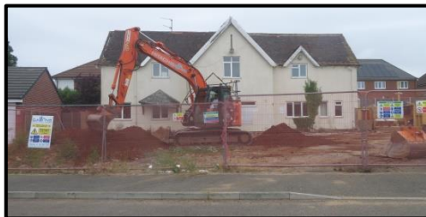
Start of demolition, 4 th July 2023.
