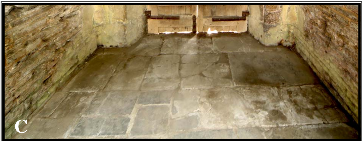
Headstones lying flat around the perimeter of the churchyard [A], some of those face up are unreadable [B] and others were used to create a floor for the porch [C].
