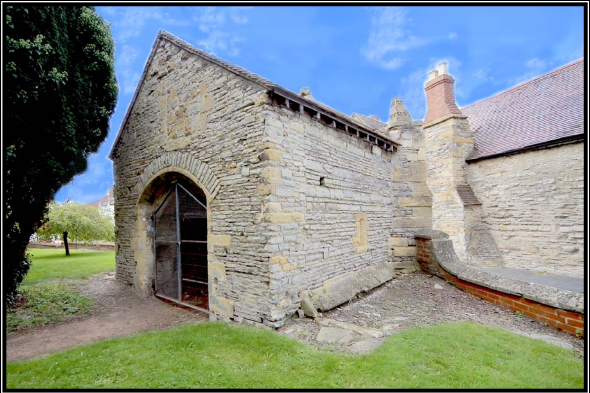
Views of the porch showing part of the original surrounding wall and the more recently added secure gated rear entrance.
